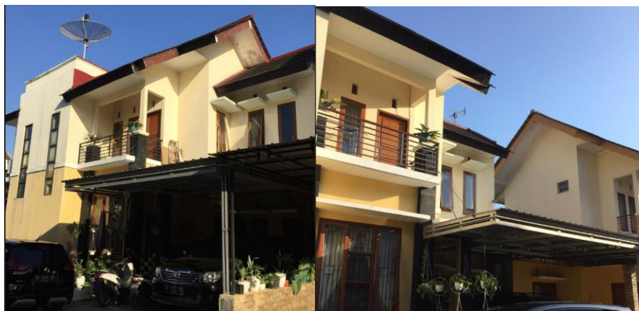
Gambar 11. Foto Eksisting Project-02 Sumber : Data Project-Architama Indonesia, 2020
