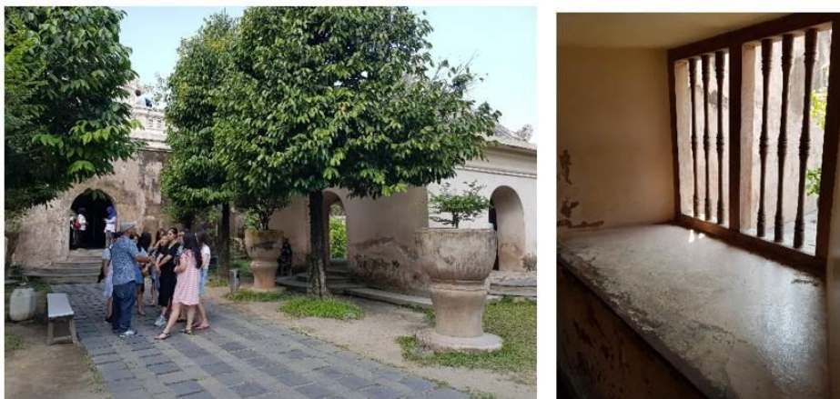
Figure 6. Activity in Gedhong Sekawan (left); wall thickness of the building (right)
