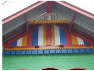
Figure 4. Ventilation ( pepir ) and ornaments on the top of the exterior
