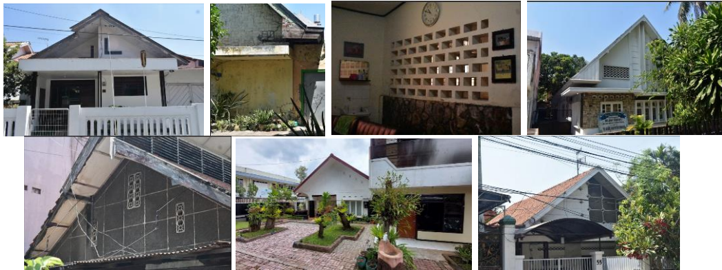
Figure 9. The use of ventilation blocks ( rooster ) arranged linearly on the building façade Source: Author, 2024
