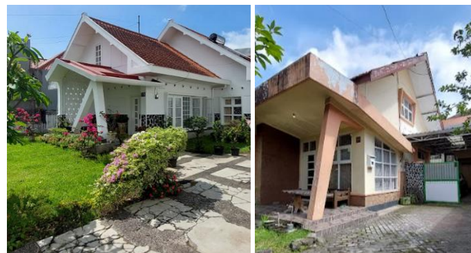
Figure 2 The front wall appears slanted (in Malang) Source: Author, 2024
