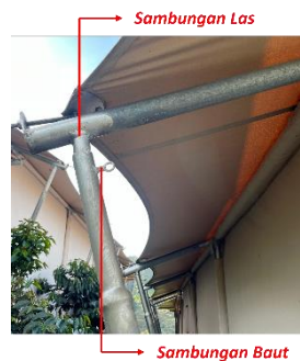
Picture 11. Identifying the Connection System on the Snail Tent by Asstro Highland (Source: Author's Document, 2024)
